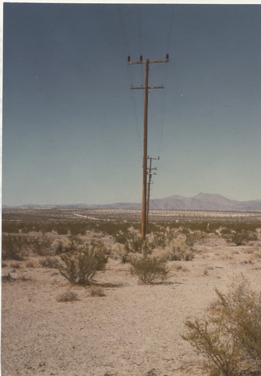
FIGURE 47. View of the 1961 epicentral region showing tilted telephone poles.
